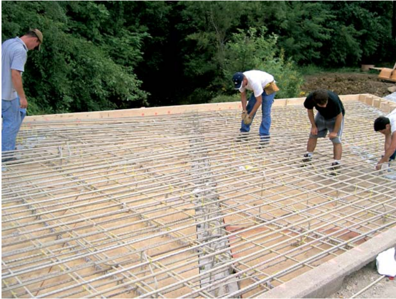
Fig. 2 Setting a FRP network for casting a construction concrete in the repair of a bridge (Courtesy of D. Gremmel, Hughes Brothers)
